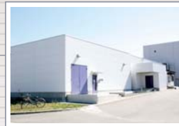
EUV-Laser Experimental Facility
