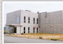
Structural Biology Experimental Facility
