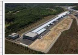
XFEL Construction Sight
